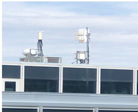
Tower on roof
